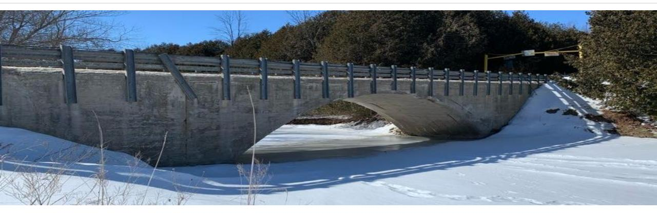
Bridge 16-WG is in an advanced state of deterioration and has been closed for public use at this time. The existing bridge is also a single-lane with other functional and operational deficiencies. Therefore, the Township of Centre Wellington has the opportunity to identify and evaluate alternative solutions and determine a preferred bridge solution in accordance with the MCEA Process.
