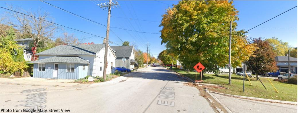
• Narrow sidewalk on north side adjacent to houses, no curb, minimal boulevard, no sidewalk on south side.
