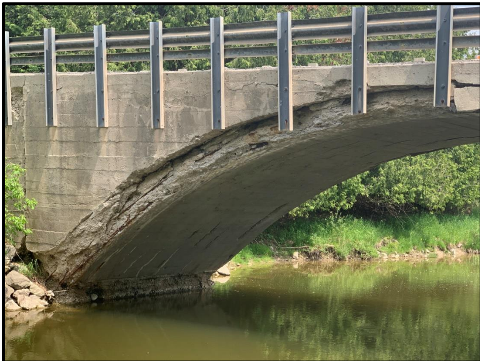
Image 14: West Elevation - Deterioration Detail Northwest Quadrant (May 25, 2021; View looking North)
