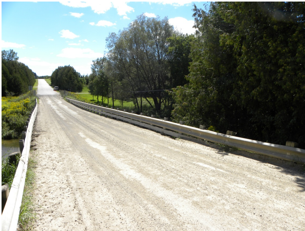
Plate 9: Bridge deck showing gravel on deck surface, and barrier railing structures
