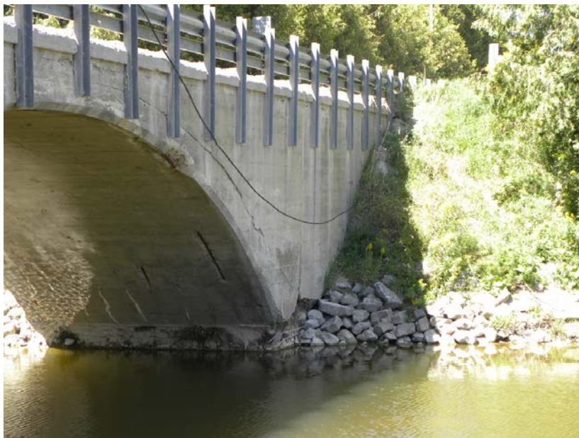
Plate 8: East side of the north abutment showing evidence of exposed re-bar in the arch soffit and stone rip-rap protection of the abutments
