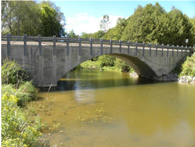
Plate 7: Upstream (east) side of the Fifth Line Bridge, showing abutments and spandrel concrete arch. The springing line of the arch is visible just about the water level on the left (south) abutment
