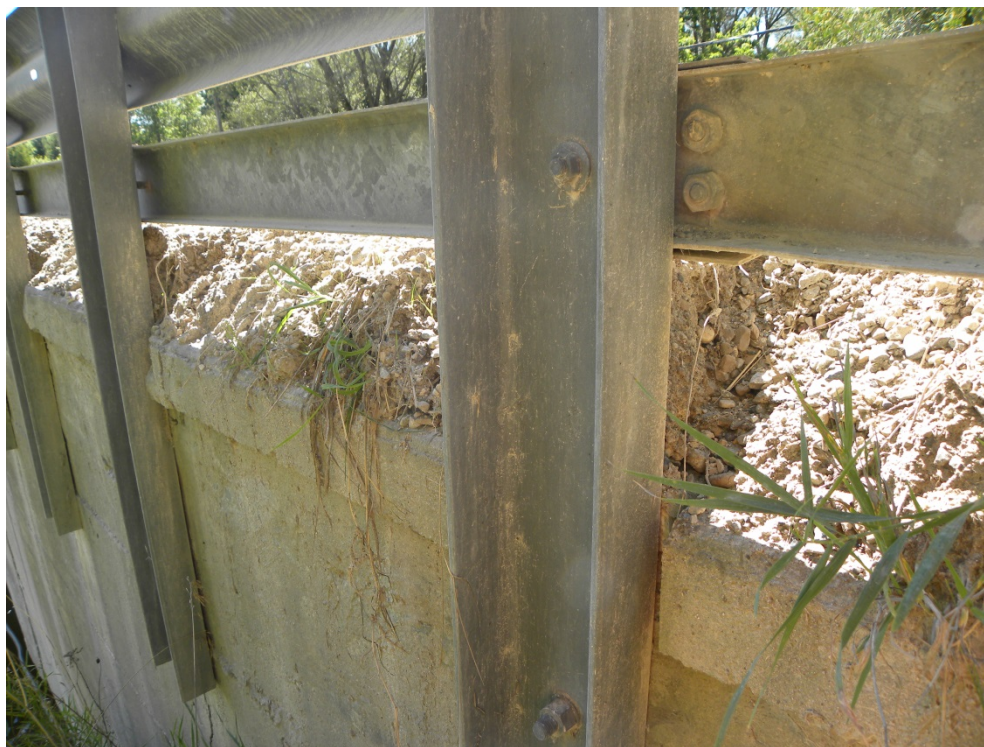
Plate 10: Post detail showing cut into spandrel wall to house post and bolt system to anchor post to structure, and deck gravel piled higher than spandrel walls.
